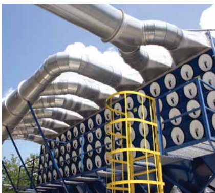
DFO on Sawdust 57,500 cfm (97,692 m 3 /h)
