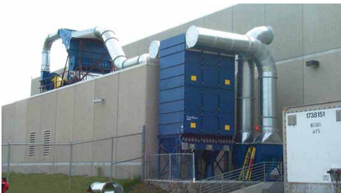
DLMC on Paper Dust 27,000 cfm (45,864 m 3 /h)
