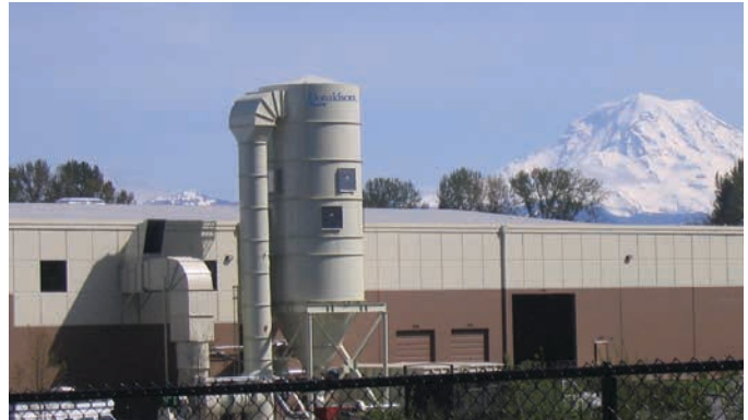
528LP12 at Cabinet Factory 70,000 cfm (118,906 m 3 /h)
