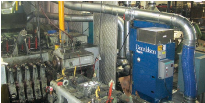
WSO on Smoke - Cold Forming 1,200 cfm (2,038 m³/h)
