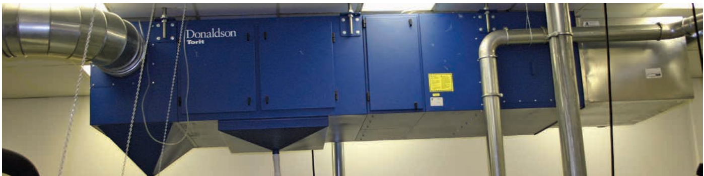
MODULAR MEDIAFILTER™ on Grinding 2,000 cfm ( 3,397 m³/h)
