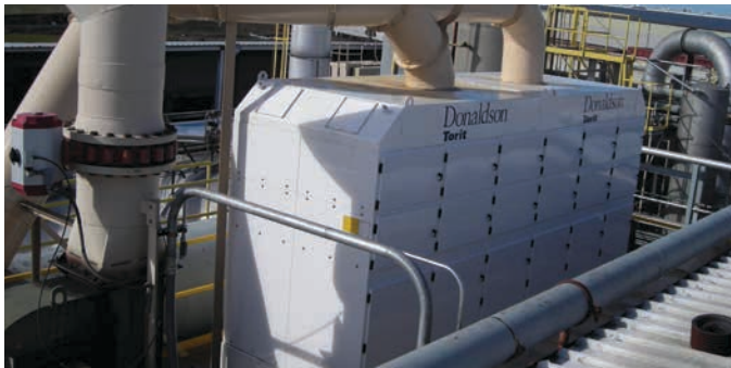
WSO on Oil Mist 20,000 cfm (33,973 m³/h)
